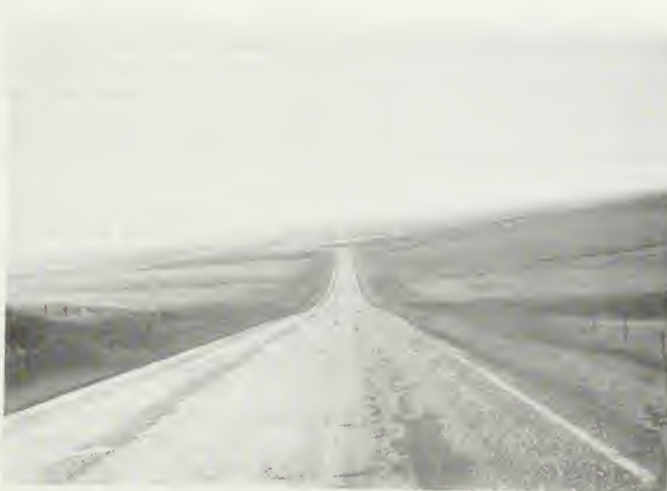
Figure 7 - South view near milepost 12.5
